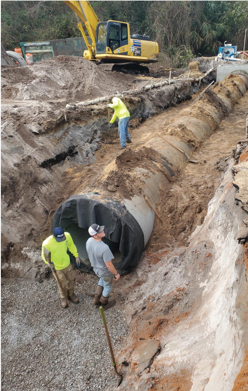
2020 East Drainage Basin neighborhood stormwater project.
