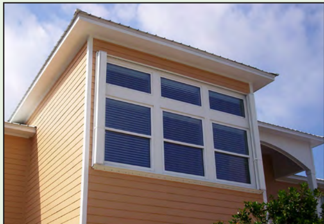
Figure 4-4: Accordion shutter (shown in the open position) installed over a large window of a coastal home. Shutter has been installed to allow deployment from inside the home. (Source: Roll-a-way/QMI)
