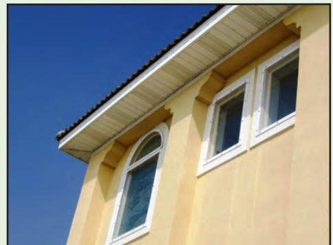
Figure 4-9: Flat impact polycarbonate panels are installed directly over windows of a coastal home. This window covering provides excellent storm protection with minimal aesthetic impact. (Source: Roll-a-way/QMI)
