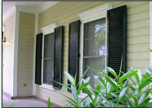
Figure 4-6: Colonial shutters made from durable extruded aluminum components add a traditional look to the home and provide effective opening protection. (Source: Roll-a-way/QMI)
