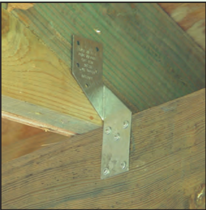
Figure 4-17: This is the popular H2.5 hurricane clip installed during new construction of houses. Five nails are hammered into the lower beam (or top plate) and five more need to be used for the roof (truss-rafter) connection. A hurricane clip is required for each truss-rafter. Upon completion of this structure, the hurricane clip will be hidden from view. This particular clip costs 30 cents. For less than a dollar in material cost, stronger ones can be installed for both new and retrofit applications.
