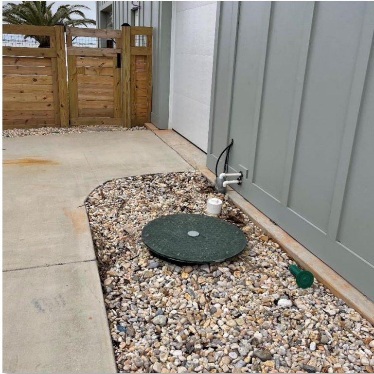
Image 3: Grinder package after installation is complete. Only the access cover is visible from the surface.
